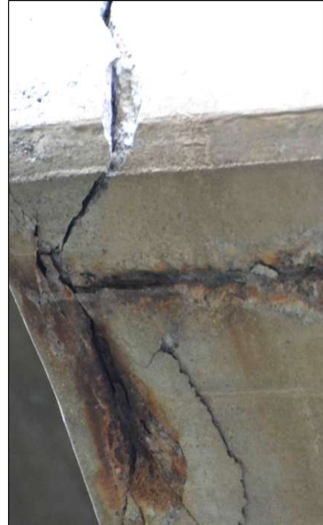
Bridge - Corrosion
