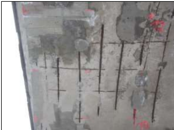
Corroding reinforcement
