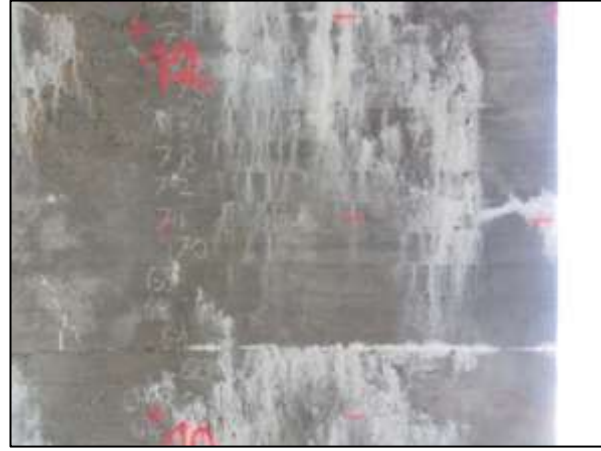
Efflorescences
